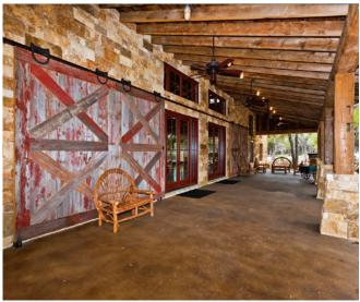
allowed us to insulate and not lose any dimensions or cut into any of the old timbers," explains Glowka. "We added custom barn wood red sliding doors that run on tracks hand forged by Amish craftsmen, and used additional reclaimed barn wood and expansive windows — all the finishing touches to make it as beautiful as it is functional."
